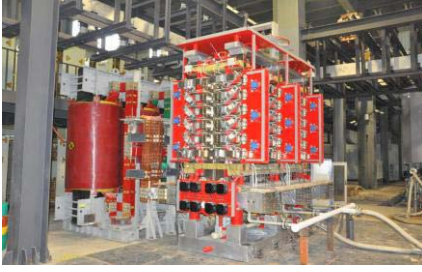
Fig. 8. Short circuit withstand test at ASIPP site.
