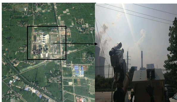
Fig. 7. Experimental site at the Feng-tai power plant.
