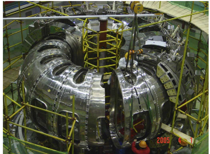
Fig. 4. Assembly of the three tori of EAST.
